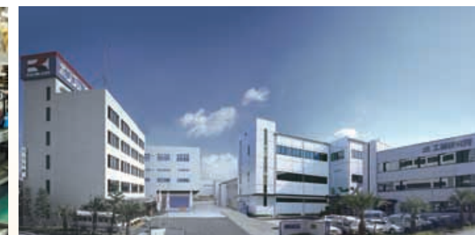
Head office and factory
